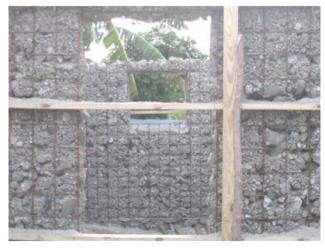
The 2012 Regional Project was to support the building of "Rubble Houses" in Haiti. These are homes that are literally built from the earthquake rubble. They cost \$4,000 each and can be erected in a week. ABCOPAD has organized several trips to Haiti to build these houses in 2011 and 2012, and more are planned in 2013.
